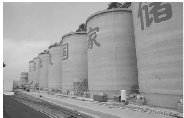
Fig. 5 Dalian Phase-2 silo block of 20 bins by 30 000 ton capacity each. The CO 2 storage-tank and ECO 2 FUME on-site mixing enclosure are dwarfed by the silos. Around the lower part of each silo is the fumigant delivery ducting.
