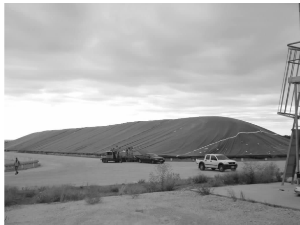
Fig. 4 A 20000-ton bunker with the HDS 800/VAPORPH 3 OS fumigation setup at GrainCorp Nhill grain storage center in Victoria Australia.
